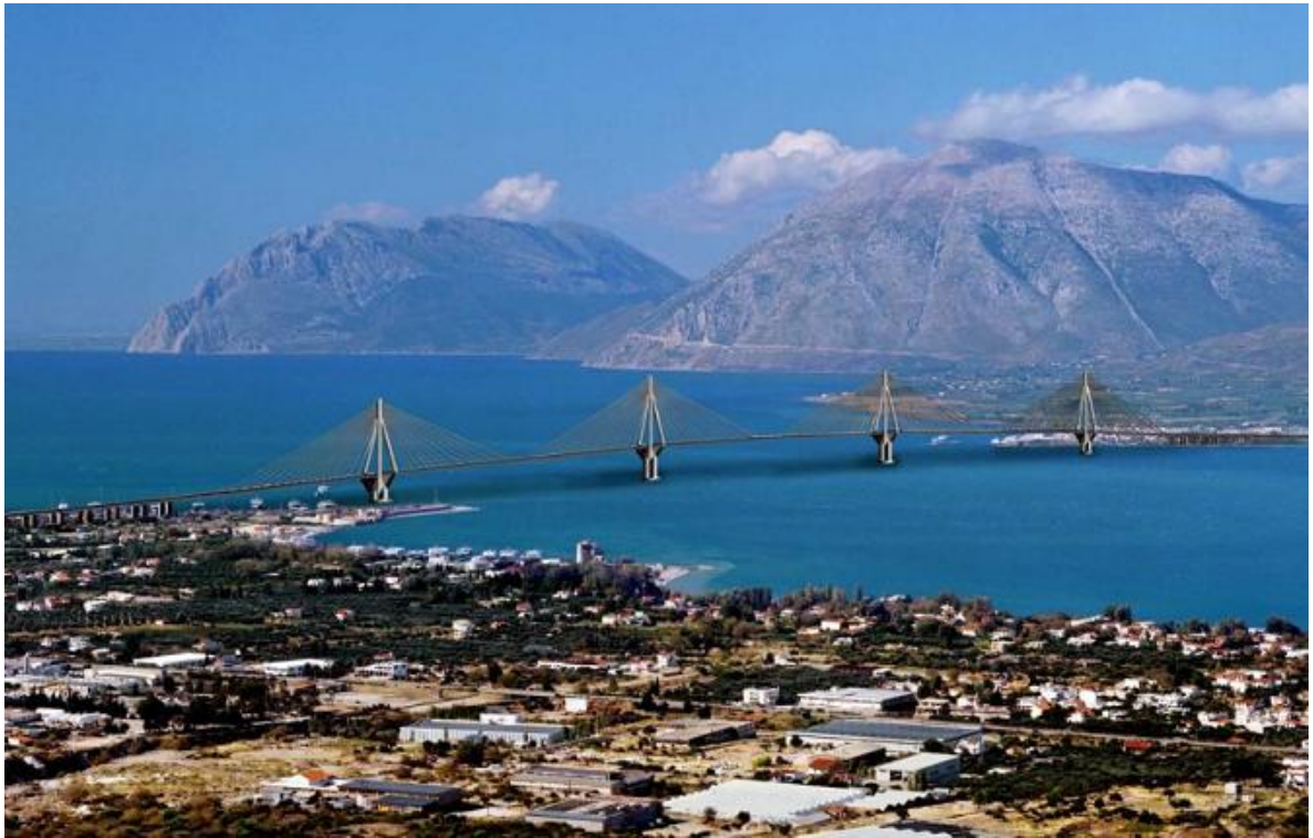
Rio Antirio bridge ( source )
